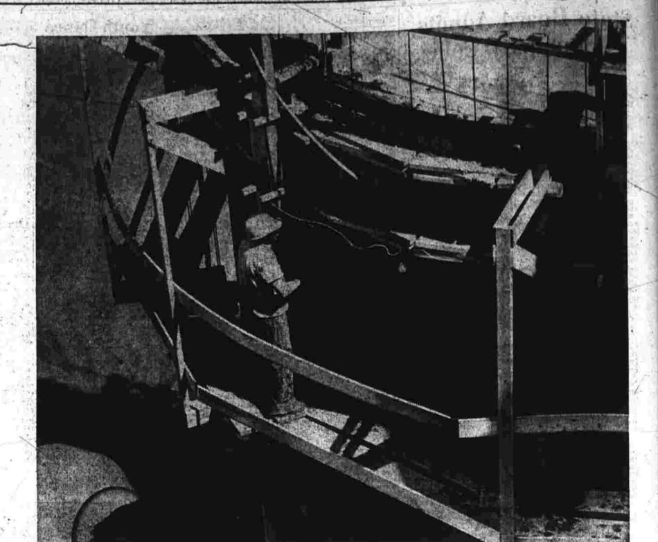
THE BIG POUR (8): The Slip Form Slips Upward, Uncovering The Concrete Still Dark-Colored In Its Curing Process
